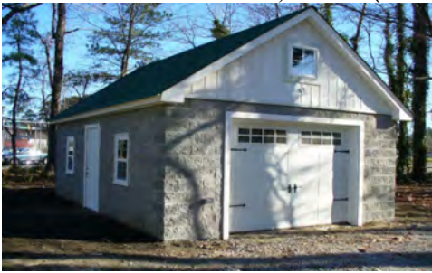
CONC BLOCK GARAGE, HALF-STORY (MS CBGH)
