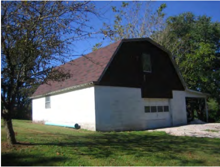
CONC BLOCK GARAGE, FULL-STORY (MS CBGF)
