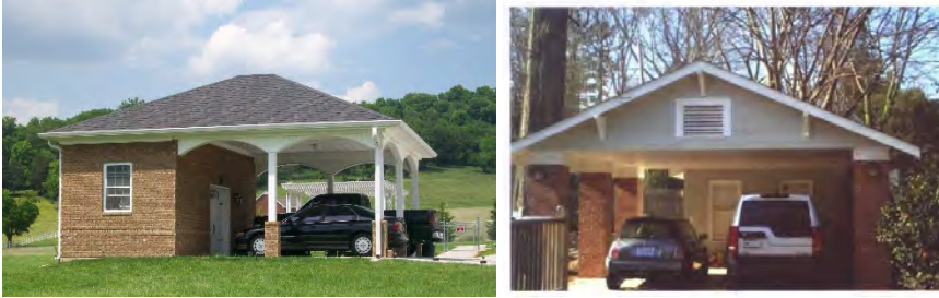
BRICK CARPORT, ATTIC & STORAGE ROOM (MS BCAS)
